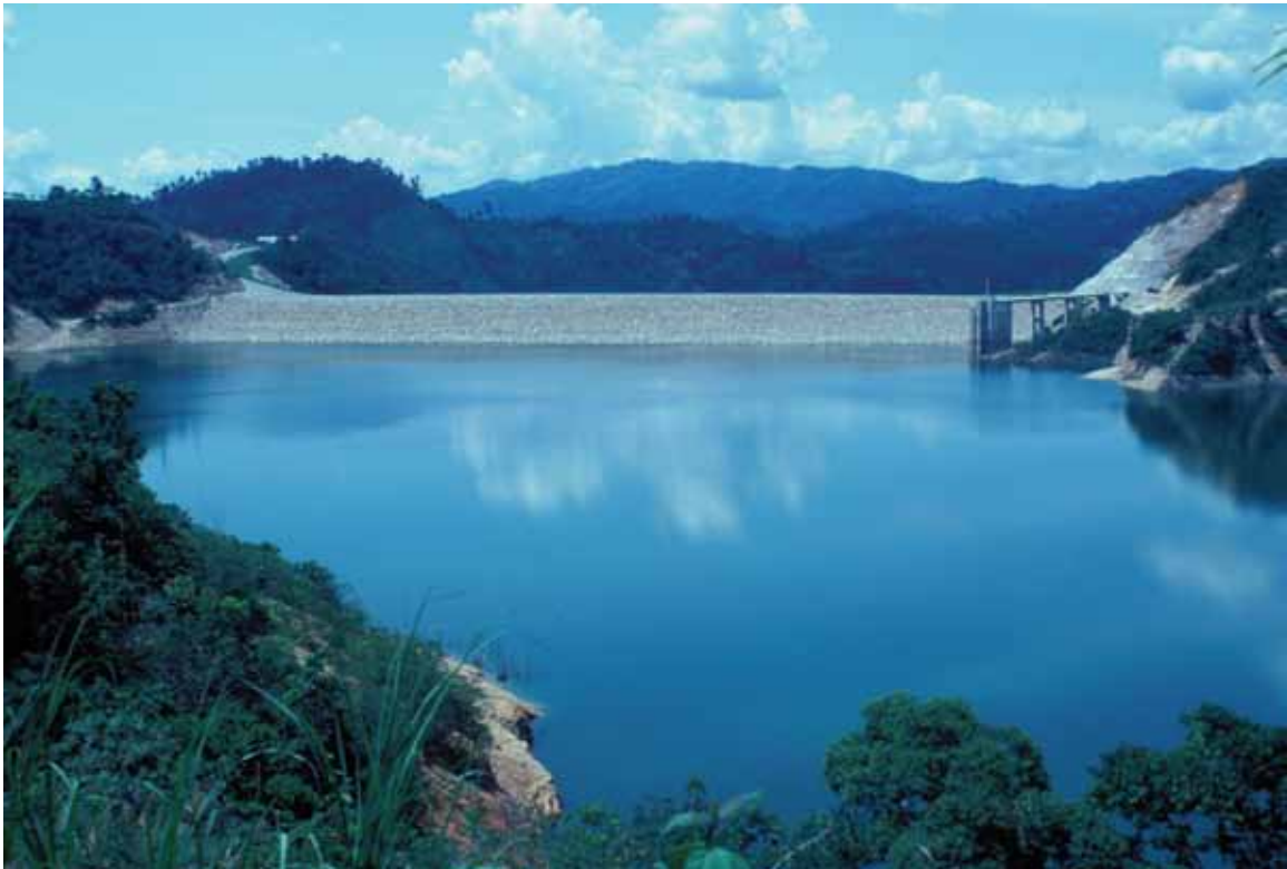
Hydropower plant in Thailand.
