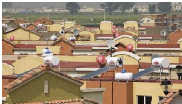
VINTE Homes: Equipped with rooftop solar panels that heat water, and natural gas cylinders that can be easily monitored and replaced
